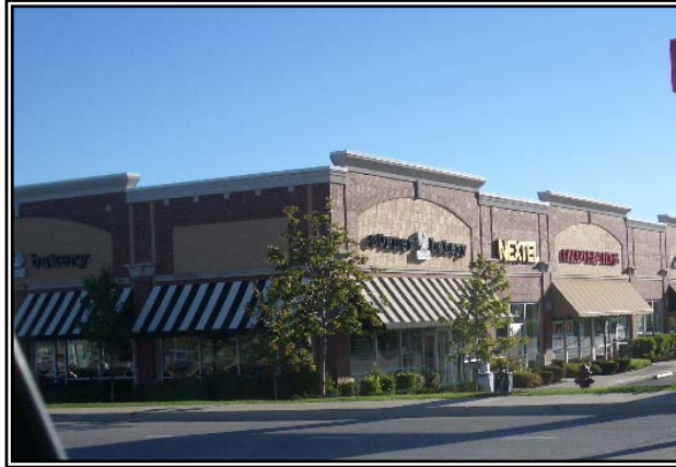
Example of outlot structure oriented towards the main thoroughfare
